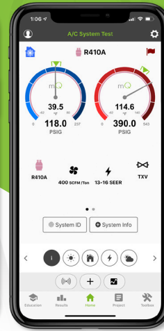
Visually Check Operation
